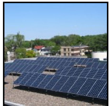
Solar Panels at Spruce Tree Centre, Part of the Energy Innovation Corridor
